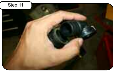
Step 11 With pliers, cut existing clamp and remove plastic elbow fitting.
